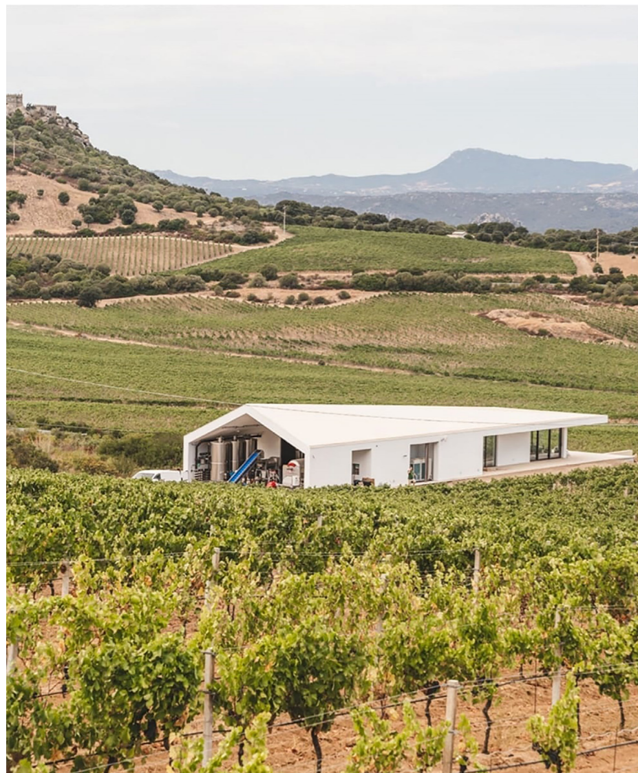
Cantina vinicola, Loiri Porto San Paolo, 2019-2021
